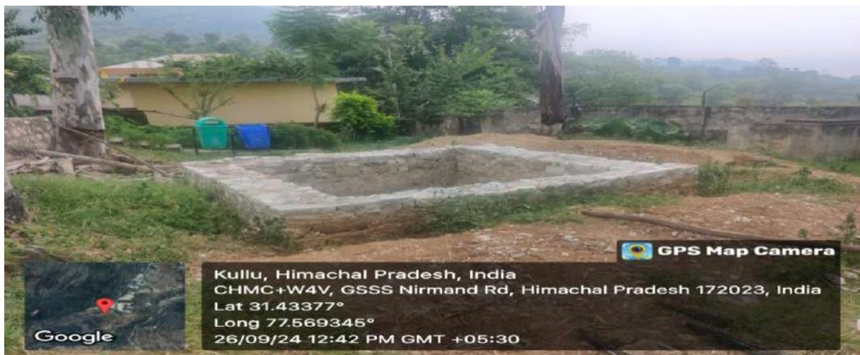
Rain water Harvesting Tank (Under Construction)
